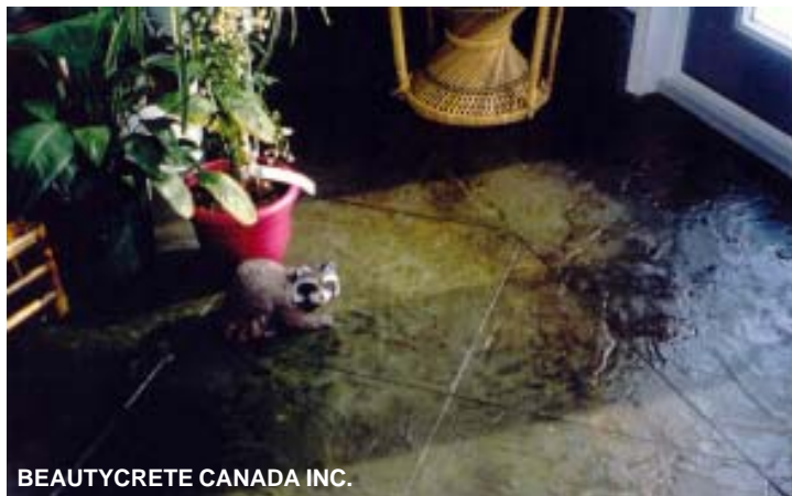
Polytop overlay stamped and then acid stained
