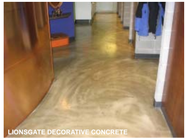
Spec-Deck overlay rough trowel finish
