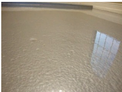
Finished Metallic Floor
