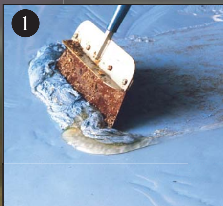
1 Scraping softened epoxy floor paint
