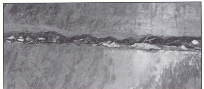
Joint deterioration is gradual but inevitable when an inferior filler is chosen or if a filler is installed poorly. As the deterioration increases, the cost of repairs increase and your productivity decreases.
