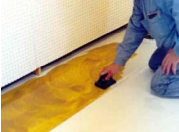
The acid stain may be applied by scrub brush, spray or any other means. Allow the stain to dry completely before scrubbing off and sealing.
