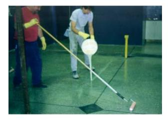
Epoxy or urethane sealers are normally used for indoor applications. Apply at 100 - 160 square feet per gallon using a low nap roller. Allow to cure for 3 days before application of the floor finish coat.
