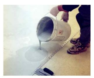
Polytop should be poured onto the surface and each subsequent pour should be placed in the wet edge to continue the flow of the material on the floor.
