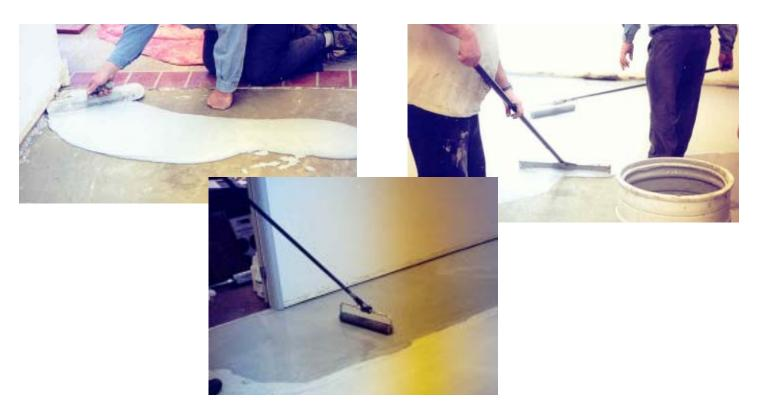
Polytop can be placed using a trowel or gauge rake to spread the material over the surface. A spiked roller can be used to remove any minor air bubbles that were created in the mixing of the product. A fresno trowel can be used to lightly finish the surface if desired.
