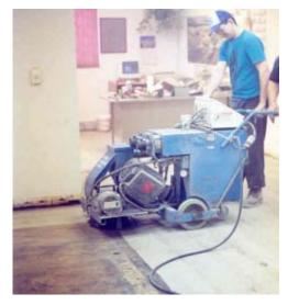
A thorough chemical or degreasing may be necessary to remove any carpet or tile adhesives from the floor. After the initial chemical cleaning, a thorough shot blasting or mechanical means of cleaning the floor is highly recommended.
