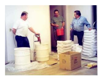
For small jobs Polytop is normally mixed in a 5 gallon plastic pail for one bag at a time or a 15-30 gallon drum where 3 - 4 bags may be mixed at a time. A mixing paddle with a 1/2" heavy duty electric drill with low speed 650 rpm is normally used.
