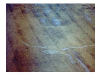
Before application of the Polytop apply primer uniformly over the substrate allow to dry clear.
