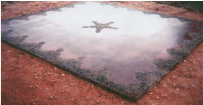
Exposed aggregate border made with the Finial pattern
