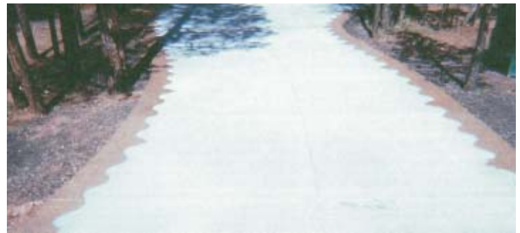
Exposed aggregate border made with the combination of Knoll and Mediterranean patterns
