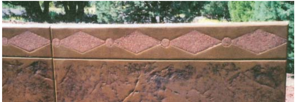
Diamond pattern exposed on a retaining wall
