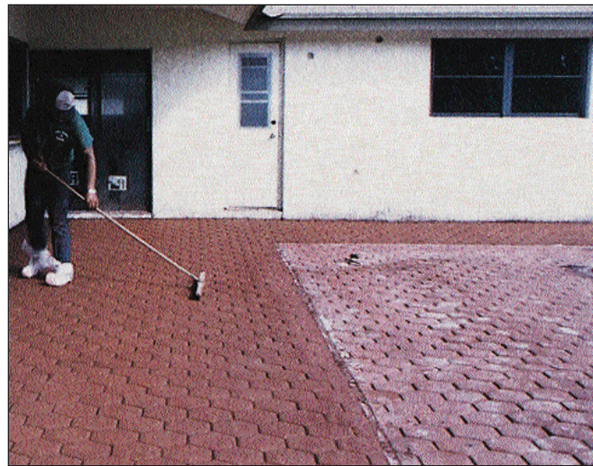
Figure 8. Wet surface brooming will remove minor stamping imperfections such as wrinkles left by the polyethylene film. Note that the worker has wrapped film around his boots to avoid marring the concrete.
