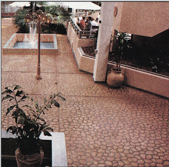
Figure 4. Deviations from straightness won't be as noticeable if long, straight grooved lines are at an angle to the line of sight and if they aren't parallel to existing walls or form lines.
