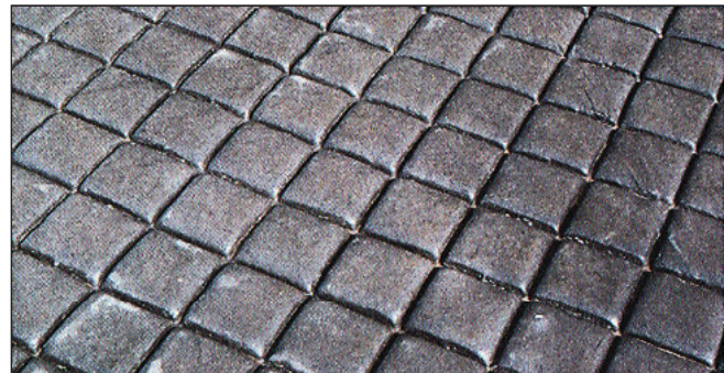
Figure 4. Deviations from straightness won't be as noticeable if long, straight grooved lines are at an angle to the line of sight and if they aren't parallel to existing walls or form lines.
