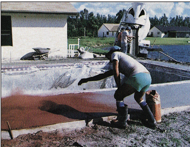
Figure 5. About half of the coloring compound is spread for the first application when no bleed water remains on the surface. Suppliers recommend using 60 pounds of coloring compound for each 100 square feet of finished surface.
