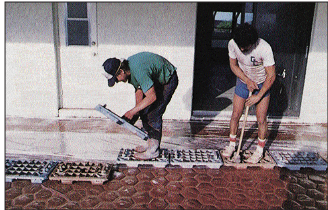
Figure 6. As concrete sets and stiffens, a sledgehammer may have to be used to produce the desired imprint depth.
