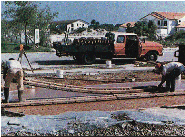
Figure 2. Plastic stamping tools can be ganged using 2 by 4's to increase production rates.
