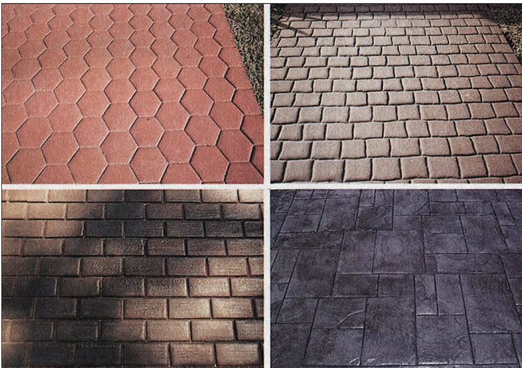
Figure 1. Four of the most common patterns are shown here: hexagonal tile, running bond brick, cobblestone and Ashlar slate. The slate pattern is made with a rubber mat, the other three with plastic or aluminum stamping tools.
