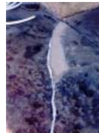
Backer rod inserted
