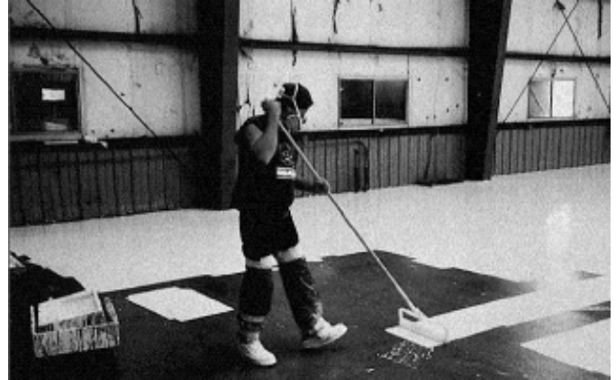
Having superior colour and gloss retention, aliphatic urethane coatings are often used where light reflectivity is important. Photo Lord Corp.
