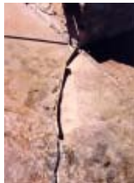
Repair done with form in place
