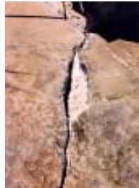
Concrete repair sawcut & cleaned up
