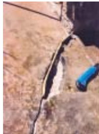
Cardboard form inserted ready for patching
