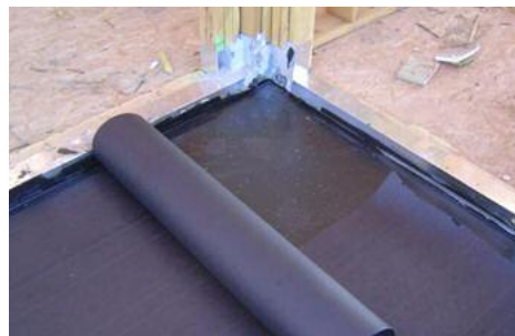
Step 3: Lay protection sheet.
