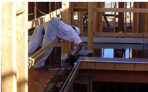
Step 1: Prime; apply EDBT; cure 24 hrs; apply 2nd coat.
