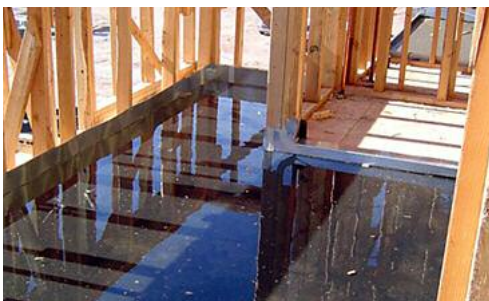
Step 2: Cure 24 hrs and complete submersion test.
